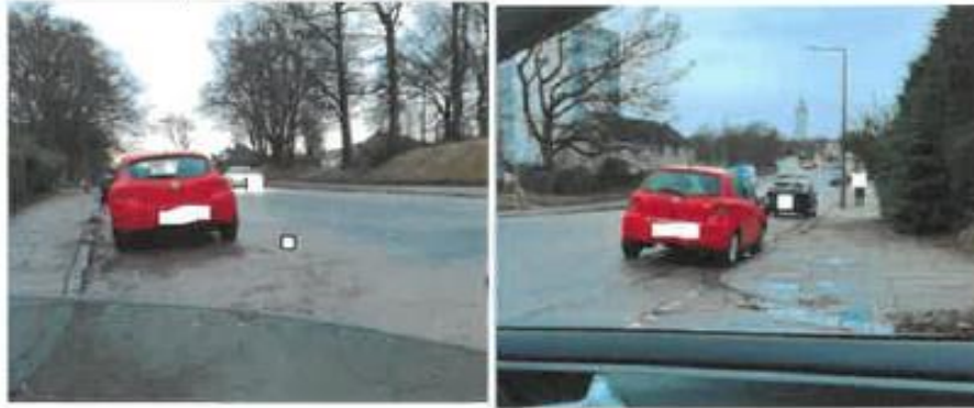
Photo 4: Hindered visibility at Middlefield Terrace – Hilton Road Intersection (4a Left: parked vehicle obstructing view of incoming vehicles; 4b Right: parked vehicles obstructing view of incoming vehicles. Note: Bus Stop at the light post). Note that it is just a coincidence that two similar red cars are parked right and left of the intersection: these are two different cars.
